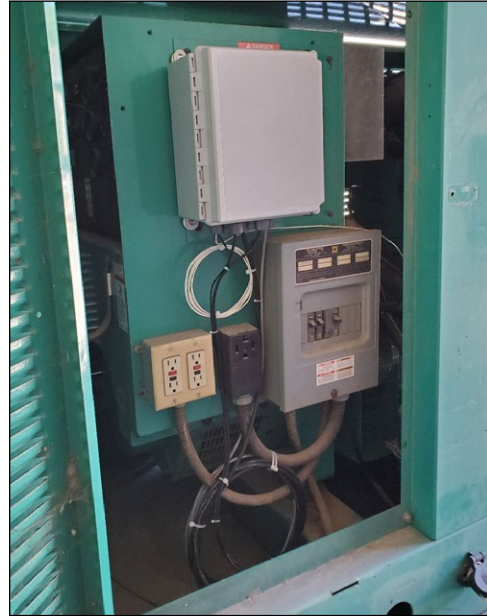
Figure 3. Solar-Powered Remote Terminal Unit Ready for Deployment
